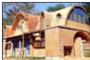
Training Centre of AV-BC With stabilised earth waterproofing
