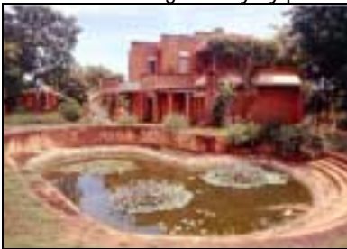
Biological wastewater treatment
