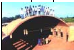
Miramukhi School 10.35 m span Built in 3 weeks
